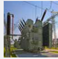
Emergency Services at 220 kV KAPCO
